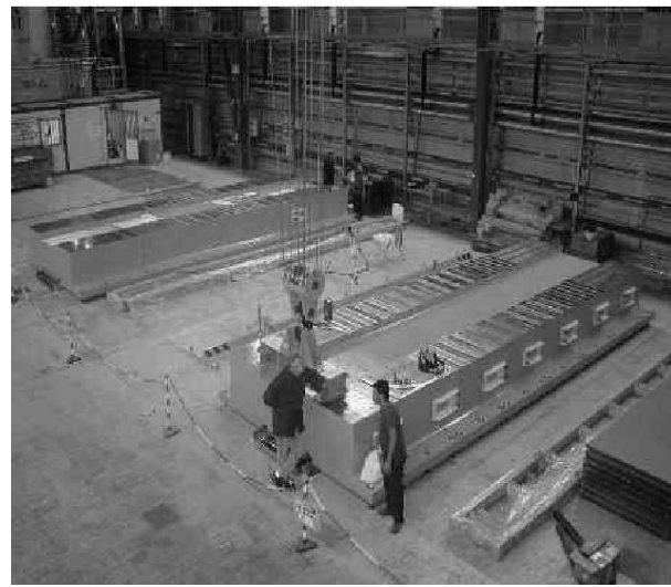
Fig. 4. The Hall C of the Gran Sasso laboratories after the installation of the bottom return yokes (Sep. 2003).
