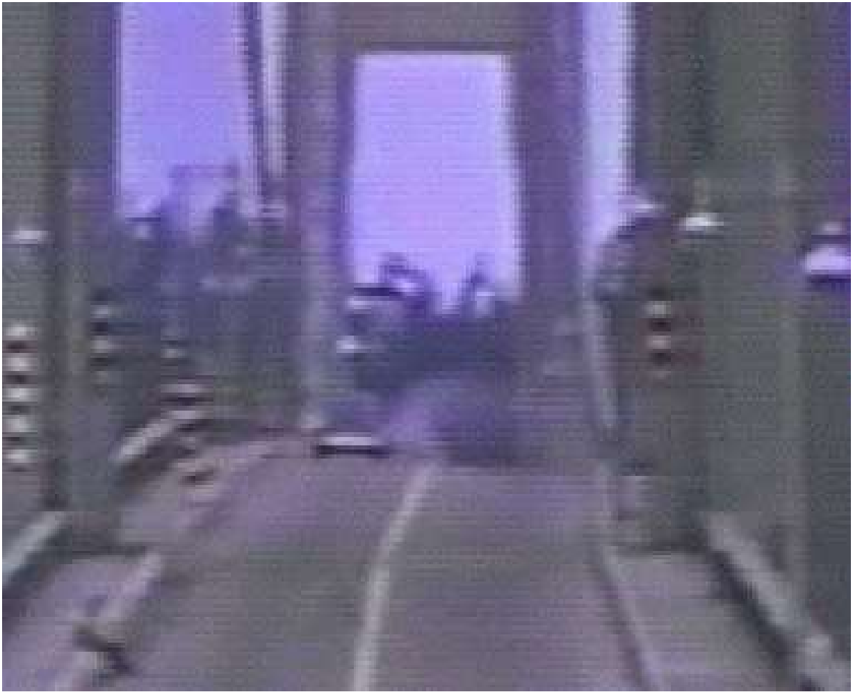
FIG. 5. Frame from the film taken by Elliot et al of the bridge collapse. To the right of the car is a large vortex outlined by the cement dust from a section of the roadway that was apparently disintegrating. To the left sits Prof. Farquarson. The behaviour of the vortex is much clearer in the film itself. The roadway is almost level in its counter clockwise rotation. Copyright "The Camera Shop". Used with permission.
