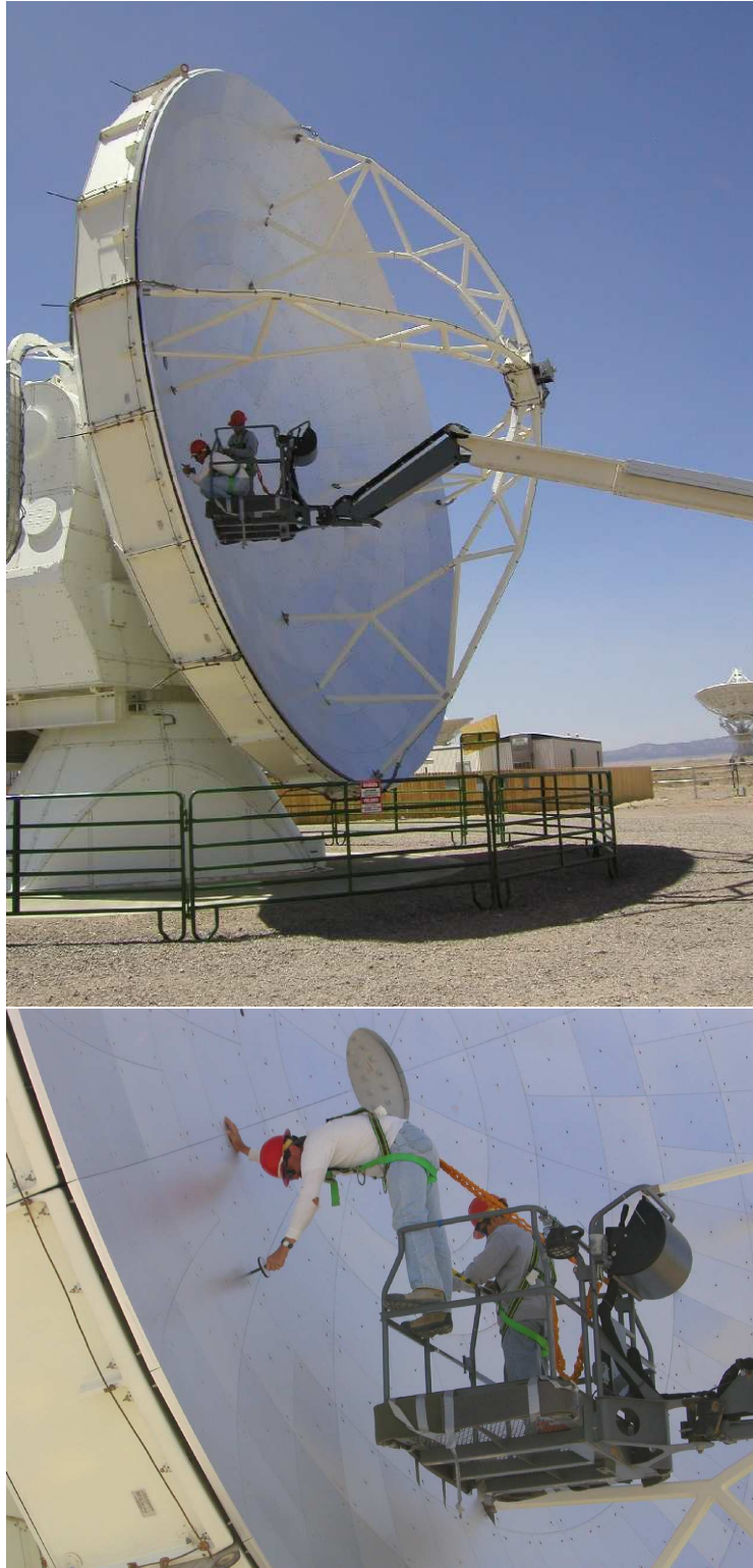
Fig. 5.— Panel adjustment of the VertexRSI prototype antenna.
