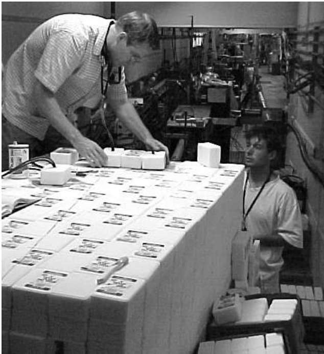
FIG. 2: View of the salt stack construction at the antenna layer. Antennas were mounted with their leads passing through drilled salt blocks as seen in several examples on the top of the stack.
