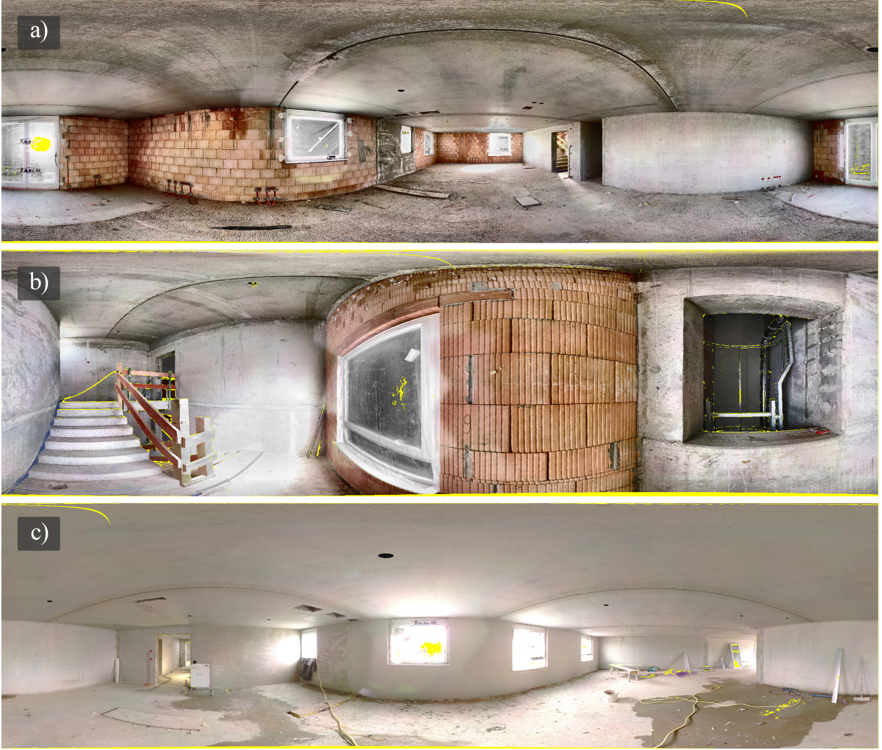
Figure 2: Spherical Point Cloud Renderings of three rooms from the custom validation dataset, collected at a residential apartment building site during shell construction. a) Medium-sized room before plastering work is completed. b) Staircase before plastering work is completed. c) Medium-sized room after plastering work is completed. The scenes are characterized by varying surface textures due to the nature of the construction, challenging lighting conditions, and complex floor plans. They include obstacles and wet spots on the floor, which produce reflections and scanning artifacts. Yellow pixels represent empty canvas pixels where no points were projected.
