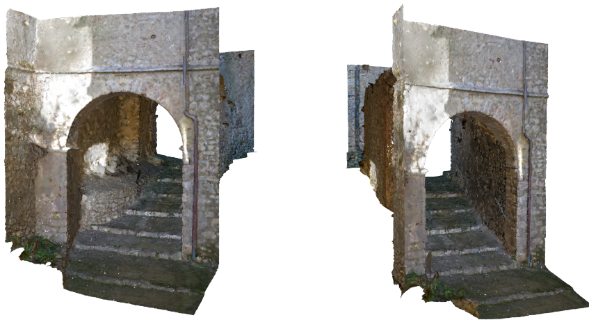
Figure 27. 3D Multi-View Reconstruction result: A scene with a stone staircase. # Face: 353K, Time: 36 min.
