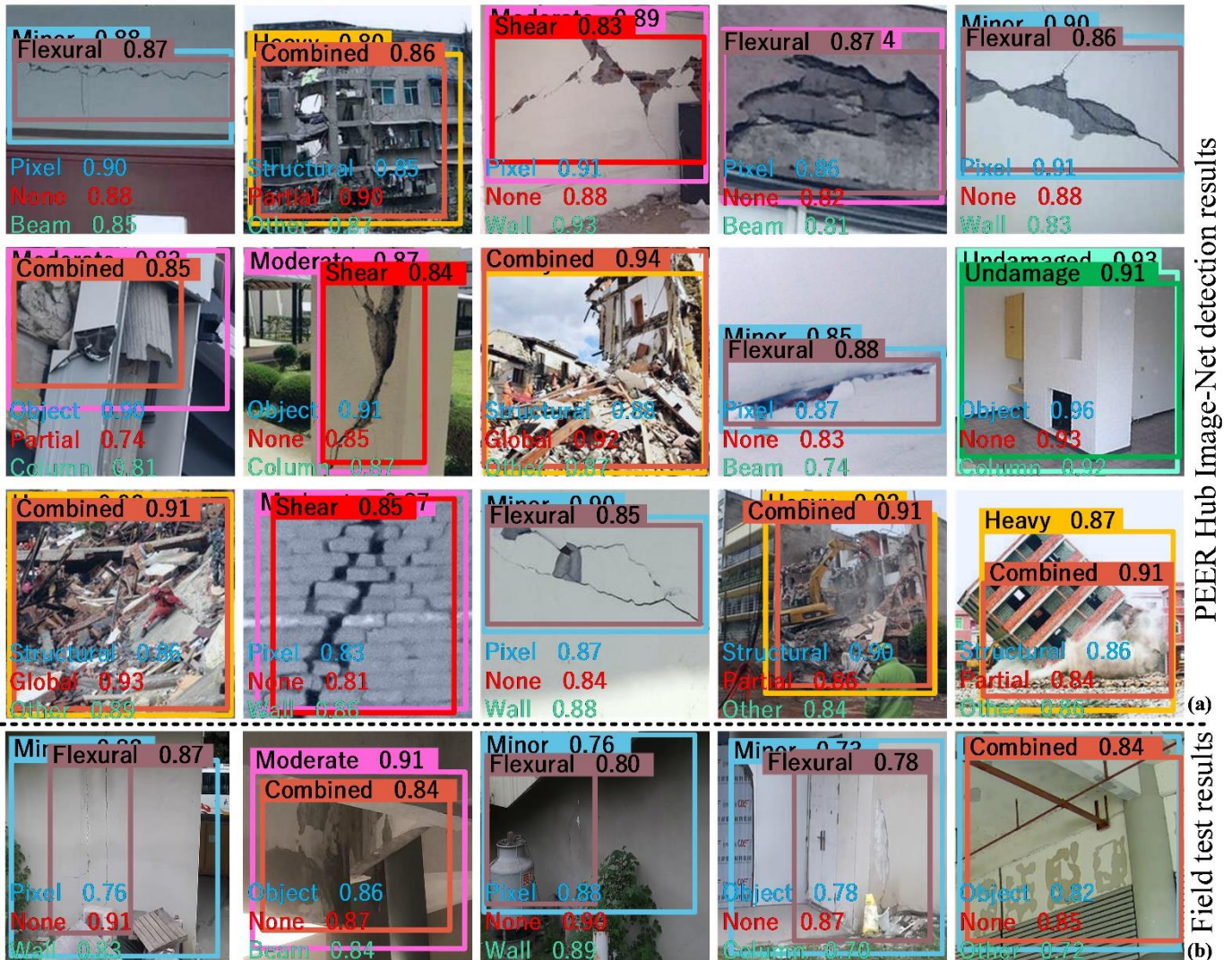
Fig. 10. Dual detection and triple classification results for Guided-DetNet: (a) results on PEER Hub Image-Net test data samples and (b) field test results.
