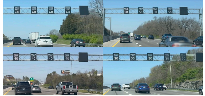
Fig. 1. The MARL-based VSL control system on I-24 Westbound: This figure shows a consecutive four gantries from a driver's perspective when approaching a congestion tail. As drivers proceed, they encounter progressively reduced speed limits of 60, 50, 40, and 30 mph displayed on each gantry, sequentially alerting them to the upcoming slow-down pattern.
