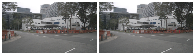
(f) left: debris; right: indicator warning board with wooden frame (15937.jpg)
