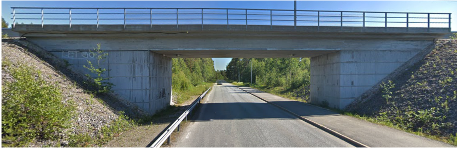
Figure 10: Hörnefors railway bridge.
