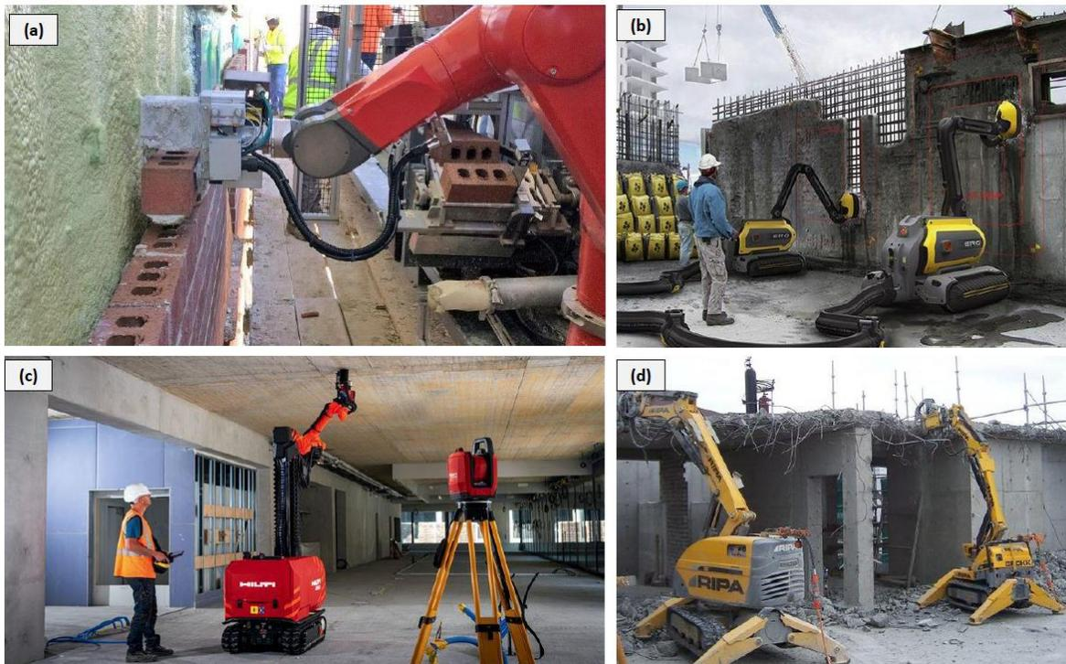
**Figure 7. Examples of application of robotics in building construction: (a) Architecture-related, façade installation (Malewar 2017); (b) Structural-related, shotcrete for shear walls (Building-Design-Construction 2013); (c) Interior layout and MEP related, BIM-**
