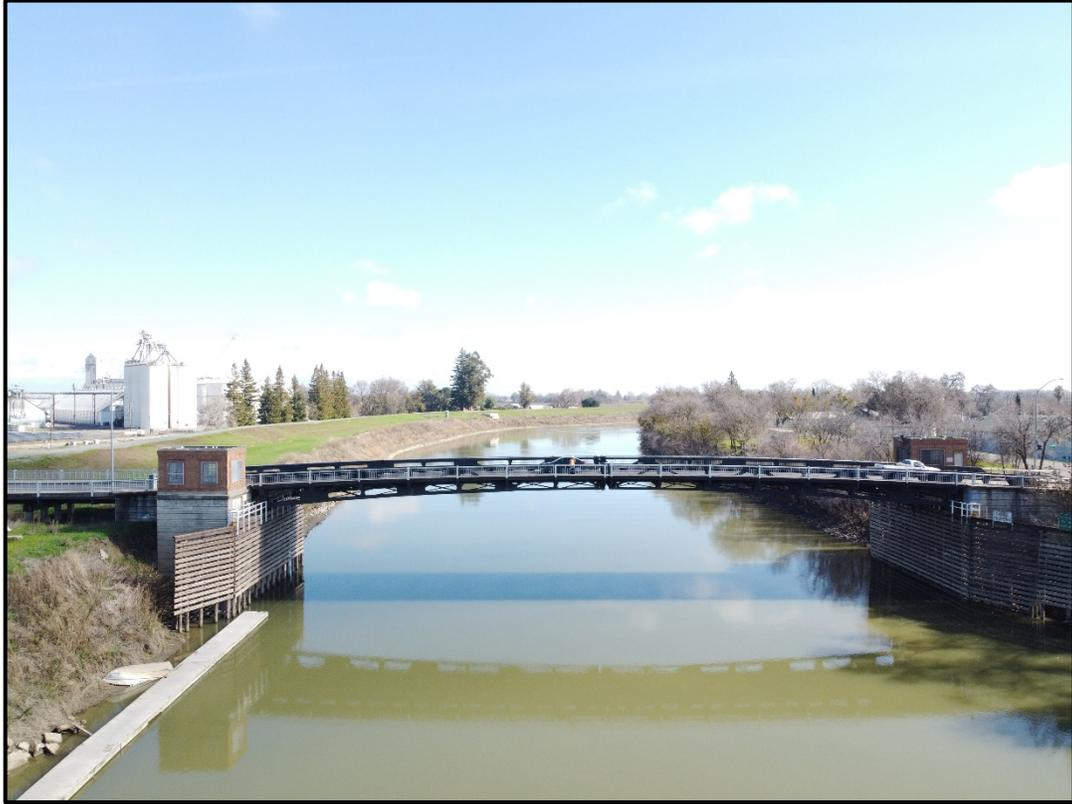
**Figure 4.** Looking downstream at the Highway 113 bridge crossing over the Sacramento River at Knights Landing, showing piers protected by timber fenders along each bank.
