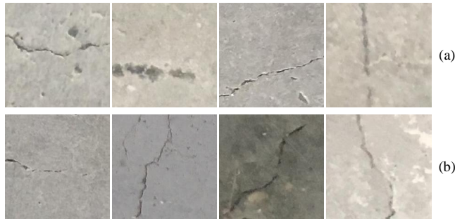
Fig. 7. The failed classification results. (a) False positive images. (b) False negative images.
