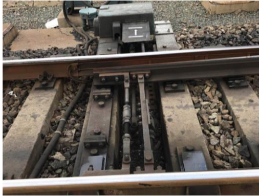
Fig. 1. Tracks moved by the turnout
