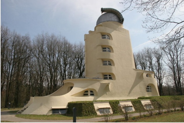
Fig. 1 North-west view of the Einstein Tower in its original light yellow-ochre color scheme. The dome is opened for solar observations. The grass covered basement contains optical laboratory, spectrograph chamber, and workshops.
