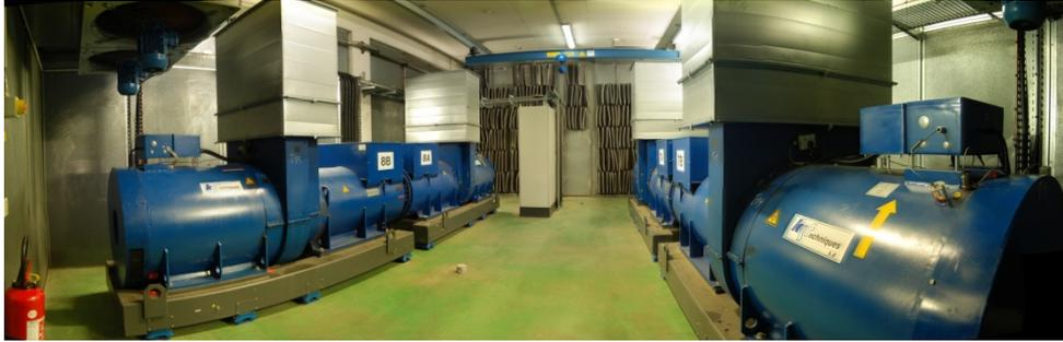
**Fig. 31:** Two twin rotablocs (four accumulators and four alternators in one cell)
