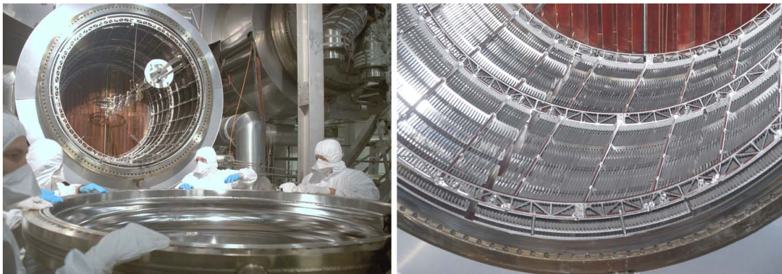
Figure 6. Left: Closing of one of the main pump ports with the NEG pump and the cryogenic baffle visible in the background. Right: A closeup view of the NEG pump with SAES St707 NEG strips installed.
