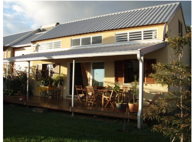
Picture 3: South West view, day part of house
