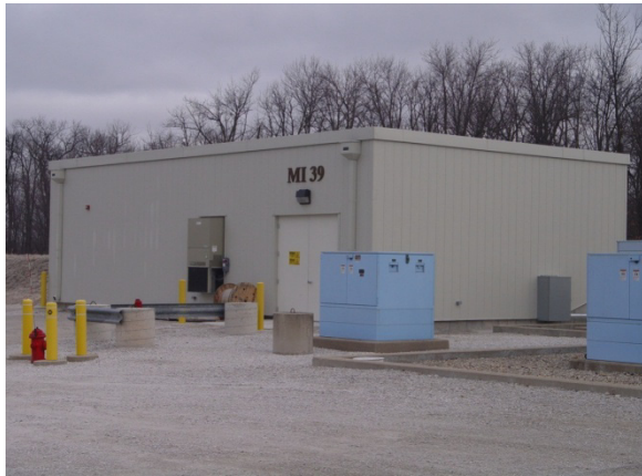
Figure 3: New kicker service building.
