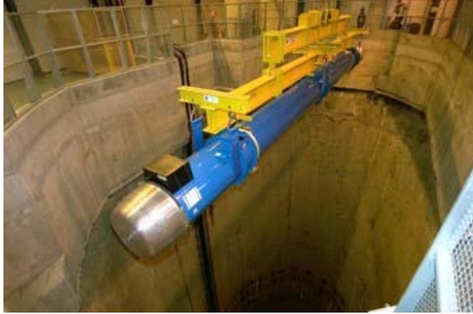
Figure 4 - Lowering of dipole into the tunnel.
