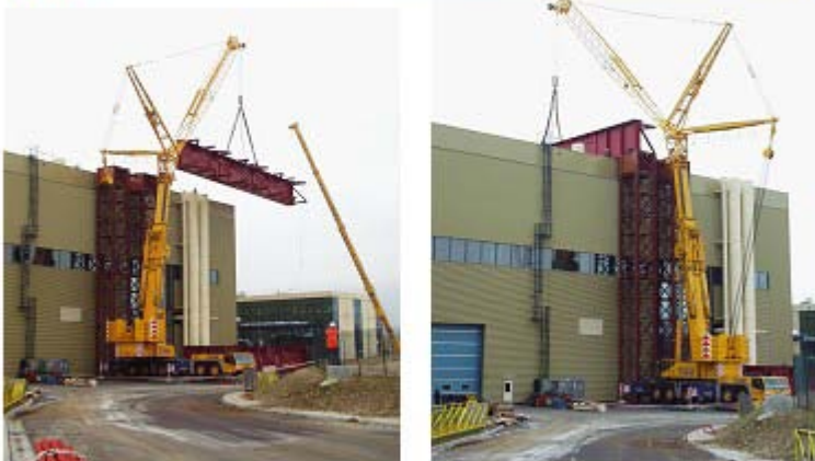
Figure 7 CMS gantry installation
