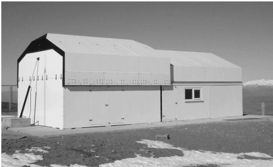
Figure 3. Reinforced glass-fiber enclosure at OAdM.
