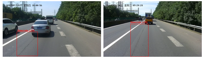
(a) Same road crack with 2.376 DetectInfo value (b) Same road crack with 4.105 DetectInfo value
