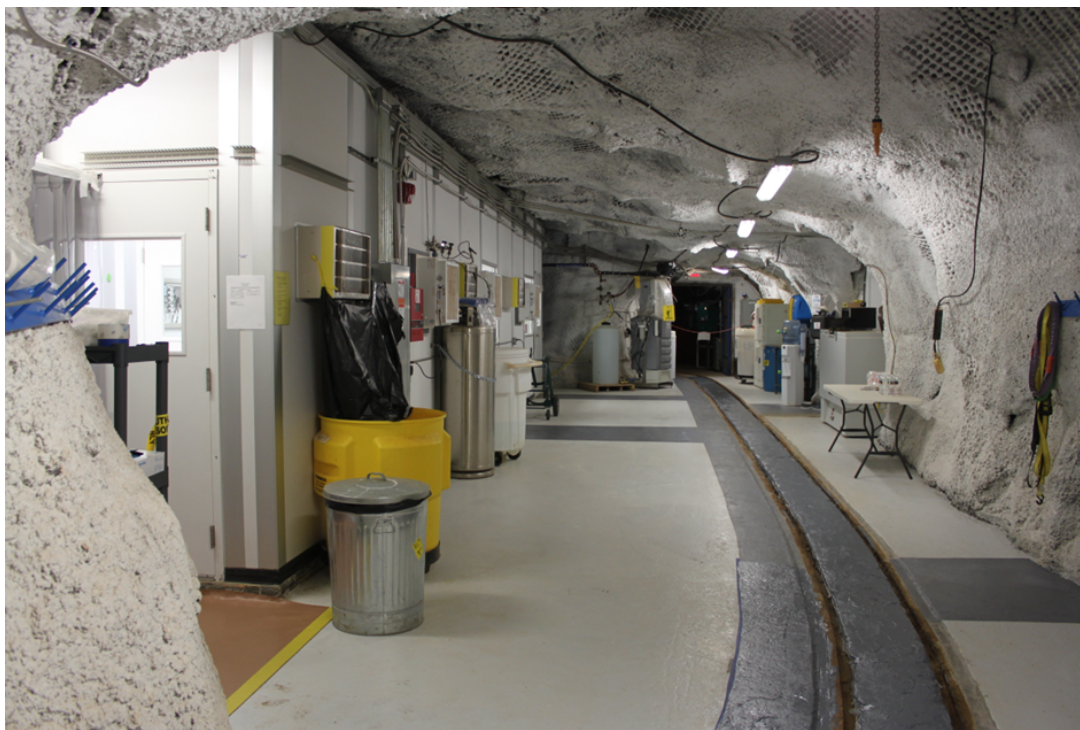
FIG. 4. The exterior of the temporary cleanroom (left), located at the 4850-foot level of SURF, at the end of its construction.
