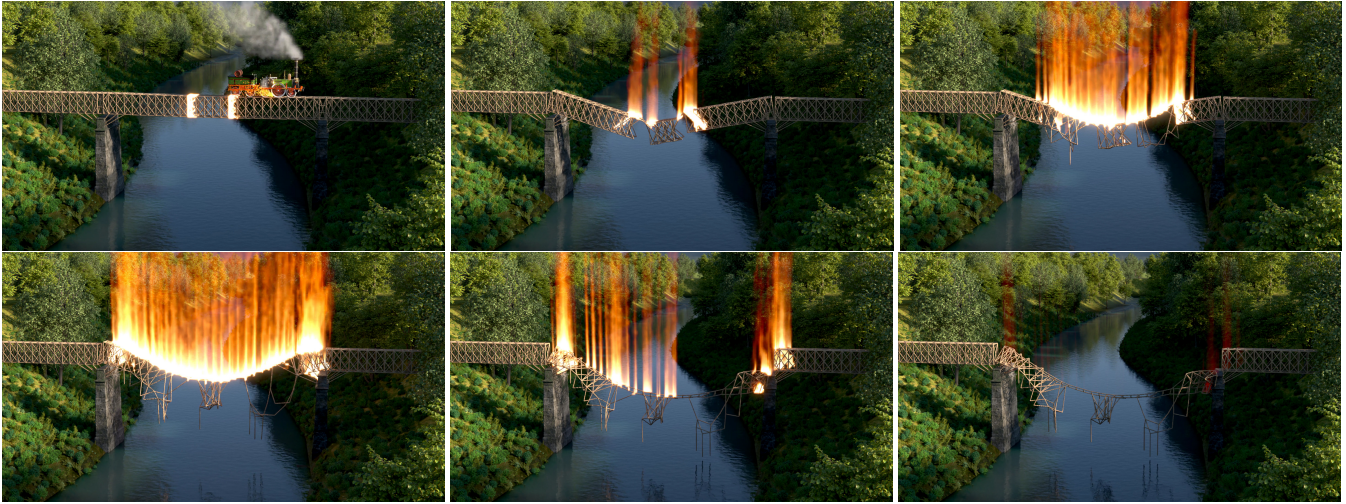
Figure 9: The historical King Louis Bridge built by Royal Bavarian State Railways (1847 to 1851) has been predominantly constructed from wood (larch, oak, and pine) as well as from iron and stone. This historical landmark of civil engineering – the oldest surviving bridge erected by William Howe – has originally been encased safeguarding the wood from glowing pieces of coal that might have fallen from locomotives for fire protection. We model such a scenario showcasing the capabilities of our FLAMEFORGE simulator. Glowing fragments fall onto railroad ties, sparking two fire sources (top row, left). The fire intensifies causing strong deformations and the characteristic sagging effect can be observed (top row, middle and right). The fire further intensifies (bottom row, left) until it can eventually be extinguished (bottom row, middle). As the fire is almost extinguished, the bridge’s central element has been severely damaged while the tracks are finally drooping in the form of a catenoid (bottom row, right).
