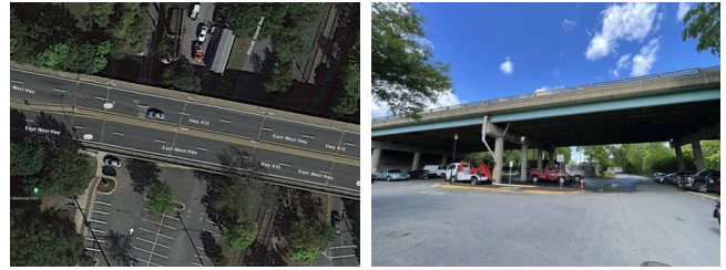
Fig. 9: Left: Google Earth image of College Park Bridge. Right: Ground View of College Park Bridge.
