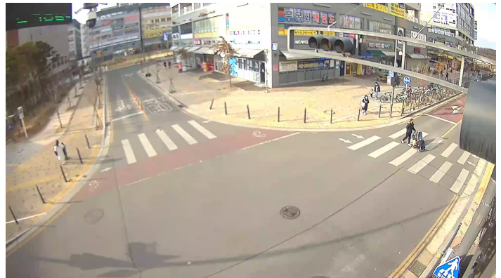
(b) CCTV Camera View of the Target Intersection
