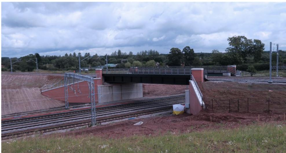
Figure 1: The IB5 Norton bridge, a composite structure with steel I-girders and a *cast-in-situ* reinforced concrete deck, spanning 26.8m
