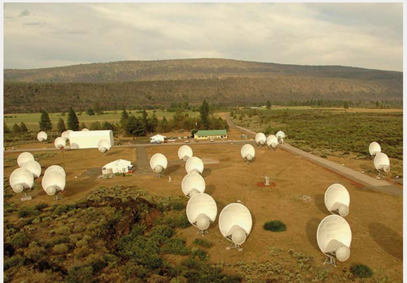
A2 Aerial view of The ATA located in Hat Creek, California, USA. The longest baseline is 323m. This array has recently recommenced observations of astrophysical transients in parallel with a SETI programme. The ATA is operated by the SETI institute. (Seth Shostak/SETI Institute)
