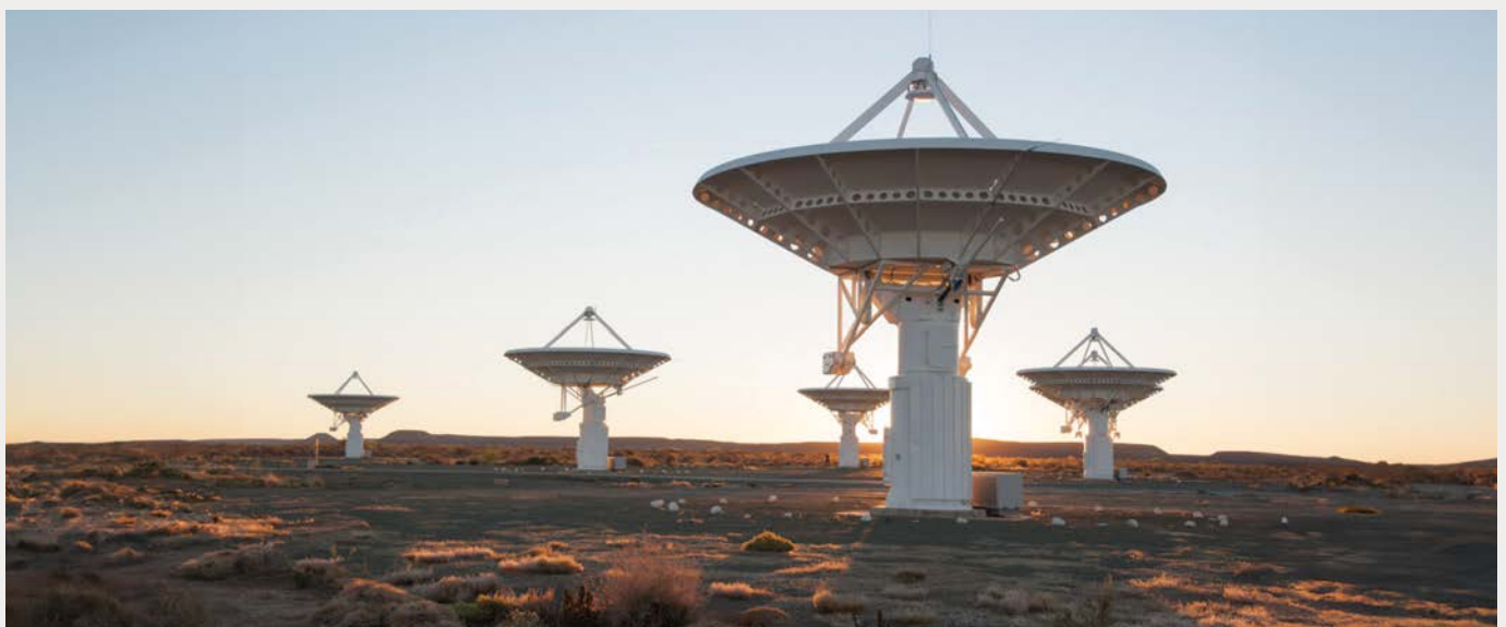
A3 Antennas of the KAT-7 array located near the MeerKAT (soon to be SKA1-MID) site in the Karoo, South Africa. The longest baseline is 185m. KAT-7 is operated by the South African Radio Astronomy Observatory, SARAO. (SARAO)
