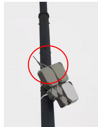
FIGURE 20: Loose external antenna and misalignment after a few months of deployment, causing connectivity problems.
