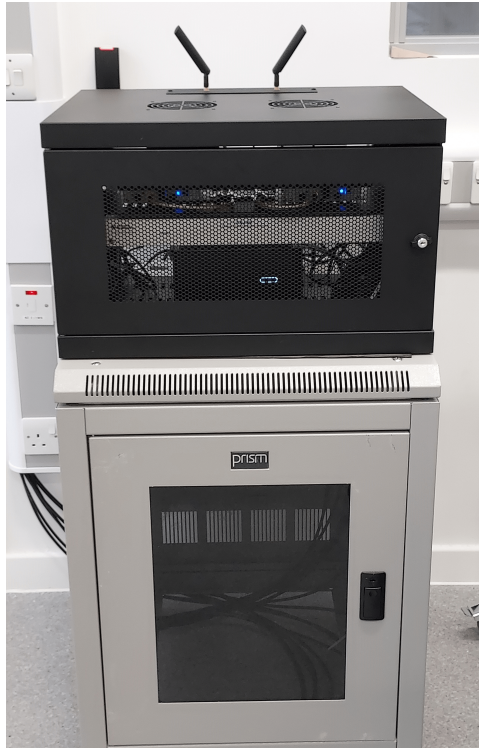
FIGURE 31: One of the 5G network-in-a-box solutions deployed in UWE (RIF).
