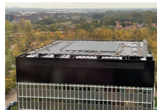
▲ As our infrastructure is modernized, ensuring it has a naturally lower carbon footprint is a high priority. Shown are solar panels on the roof of the new SRON building in Leiden.
