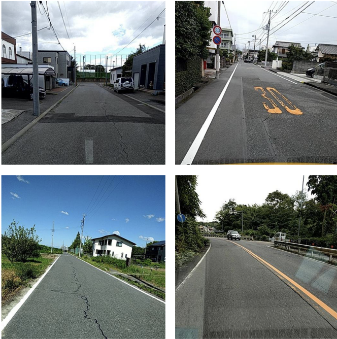
Fig. 1. Typical examples of road images collected using cameras placed on car dashboards. These images have typical perspectives. Road damages are more at the lower half of the images, and road damages may look different when they are at different positions on the images.
