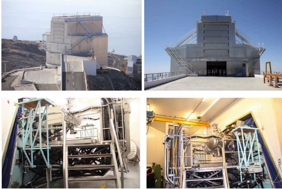
Figure 3. The telescope and the Nasmyth-A room @ NTT ESO-La Silla with SOFI, the instrument that will be replaced by SOXS
