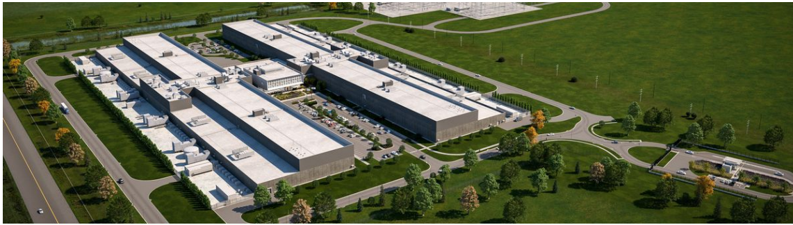
Fig. 1. Depiction of Meta's data center in DeKalb, IL, USA where low-carbon concrete discovered by artificial intelligence methods has been tested.
