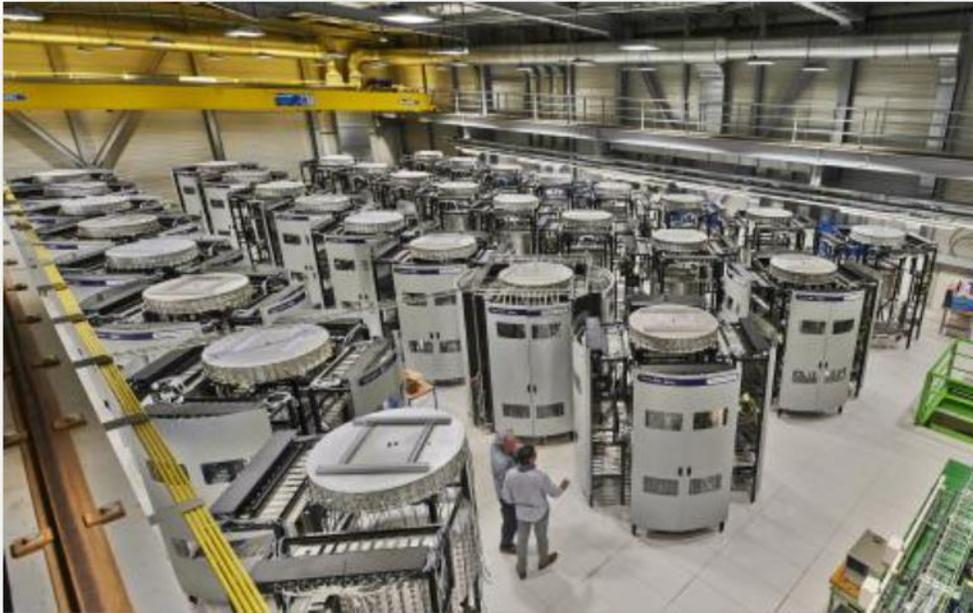
*Figure 3* CERN SPS Thales Solid State Power Amplifiers, 32 towers x 144 kW @ 200 MHz, combined into 2 x 2 MW amplifiers, into operation since 2021
