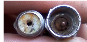
(b) Loosely tied F-connector (partly due to corrosion)
