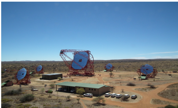
Fig. 8. H.E.S.S. IACT array at Gamsberg in Namibia, consisting of four 12 m diameter and one 28 m diameter telescope. Picture courtesy : H.E.S.S. collaboration.
