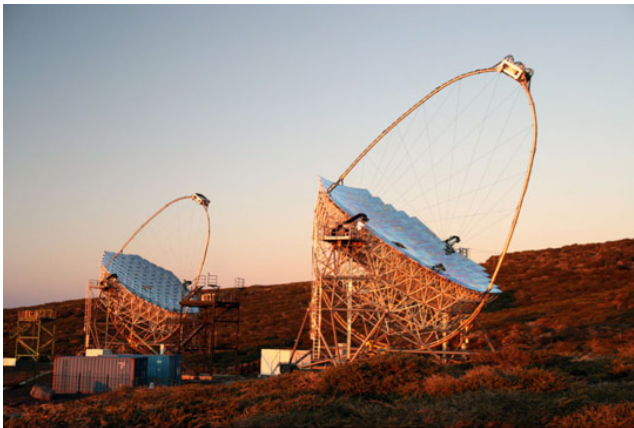
Fig. 10. MAGIC telescope system at La Palma in the Canary Islands consisting of two 17m diameter telescopes. Picture courtesy : MAGIC collaboration.
