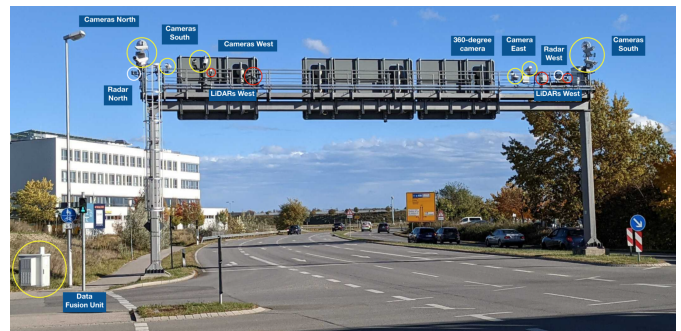
Fig. 1. An equipped intersection in the Intelligent Transportation System of the project Providentia++.
