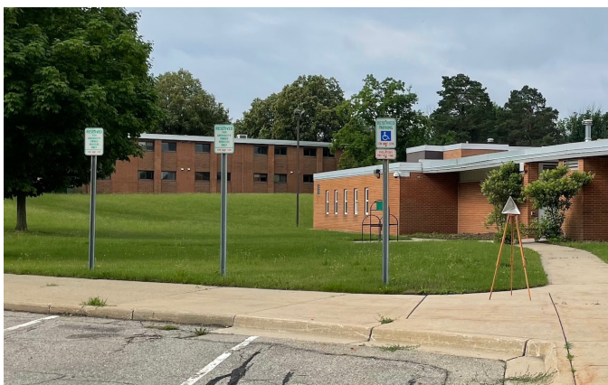
Fig. 7. Ground-based image of the row of parking signs and corner reflector used for calibration as well as the metallic exhaust chimney highlighted in ROIs 1 and 4 of Fig. 6. The cylindrical exhaust chimney is located on the roof of the building in the upper right of the image.
