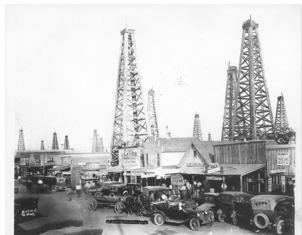
Figure 1 - Oil Derrick Drilled Through a Store
