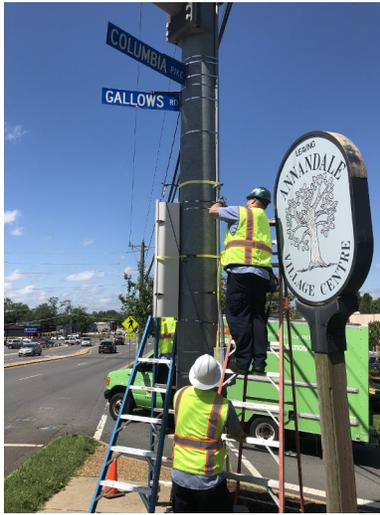
Figure 1: A typical NOVArray sensor configuration. The detector is housed in the white box and mounted to a traffic signal post.
