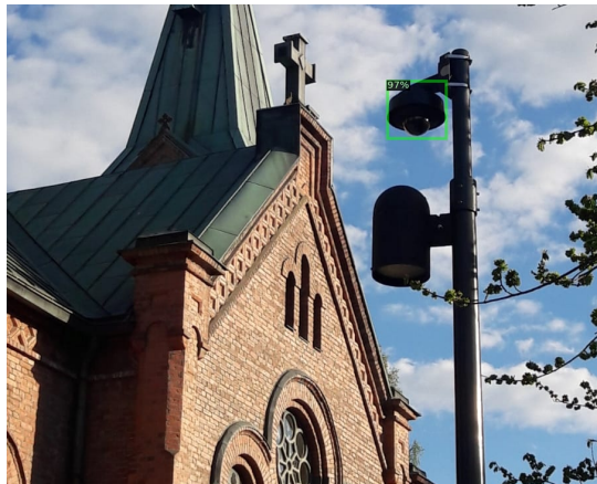
Fig. 17: Example of a hybrid installation consisting of a light pole combined with a CCTV camera. Our TridentNet model works well with a detection confidence of 97% of the “round class” instance, and avoids the potential “directed class” FP represented by the light fixture below the camera.
