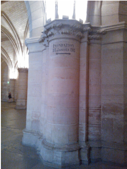
Figure 9.5: The high watermark: the level of flooding in Paris in 1910 as a maxima. Clearly one has to consider that such record will be topped some day in the future and proper risk management consists in “how much” more than such a level one should seek protection. We have been repeating the Lucretius fallacy forever.
