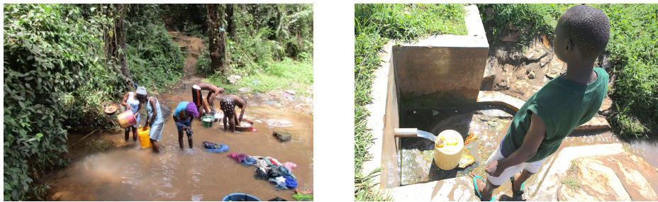
Figure 2: Images from the Busia district of Western Kenya, where 43% of individuals access water for drinking and cooking from unprotected springs (left). International Child Support, a local NGO, builds concrete structures (right) for residents to access cleaner water. From https://www.povertyactionlab.org/evaluation/cleaning-springs-kenya .
