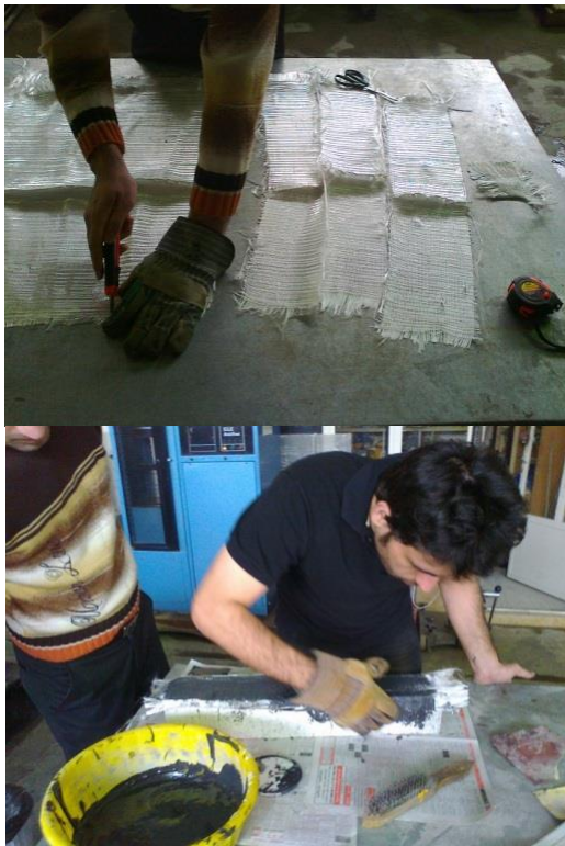
Fig. 3. Cutting and attaching the GFRP sheets
