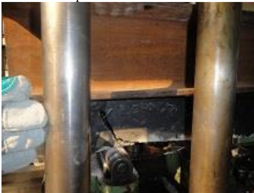
Fig. 4. Brittle failure in the distance between the two stands
