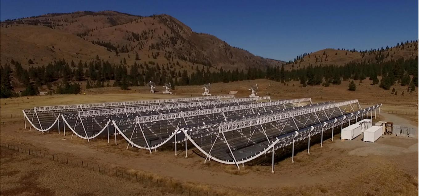
**Figure 1.** Photograph of the CHIME telescope on 15 September, 2016, looking North-West. The shipping containers housing the X-Engine and CHIME/FRB backend can be seen adjacent to the right-most cylinder. The receiver huts containing the F-Engine are beneath the reflectors and cannot be seen here. The DRAO Synthesis Telescope (Kothes et al. 2010) can be seen in the background. See Table 1 for detailed properties of CHIME.
