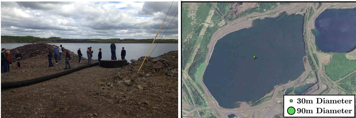
Figure 9: (Left) A photograph of the Wentworth Mine Pit. (Right) a composite satellite image of the region including roads. A cross section marker of 30 m and 90 m diameter is given for scale. Photograph courtesy J. Meier, satellite image from Google Earth.
