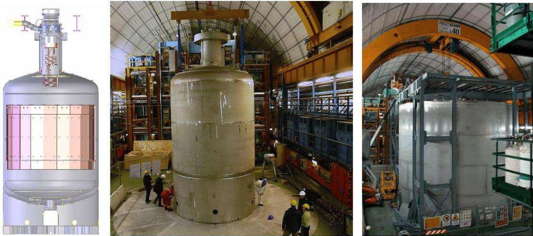
Figure 2: LAr cryostat with copper shield and active cooling system (left), the cryostat mounted on the water tank's bottom plate in Hall A (middle), and the construction of the GERDA building around the finished water tank which houses the cryostat.
